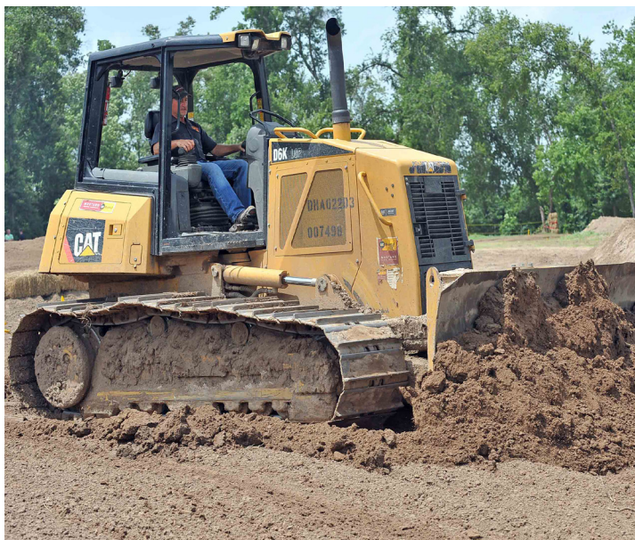
OWNER EMIL SHEBELBON PREPPING THE GP TRACK
